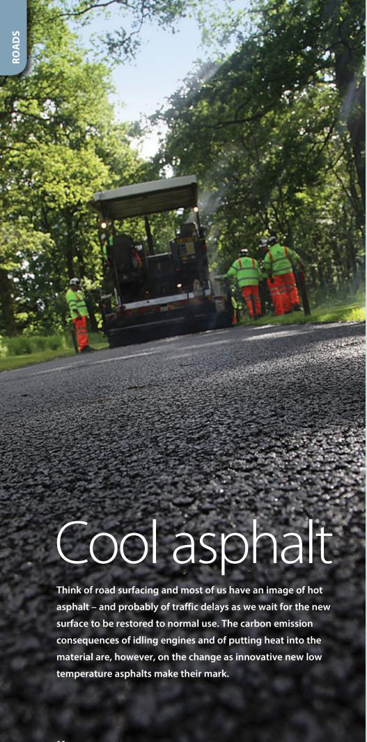
ONE of the best bits of news in the world of roads is that asphalt no longer has to be hot to be effective. It cuts carbon but it also saves precious construction time which means that roads can be back in use much more quickly. Welcome to the world of low temperature asphalt (LTA).
