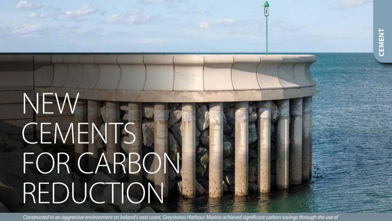
Constructed in an aggressive environment on Ireland's east coast, Greystones Harbour Marina achieved significant carbon savings through the use of concrete made with a multi-component cement
